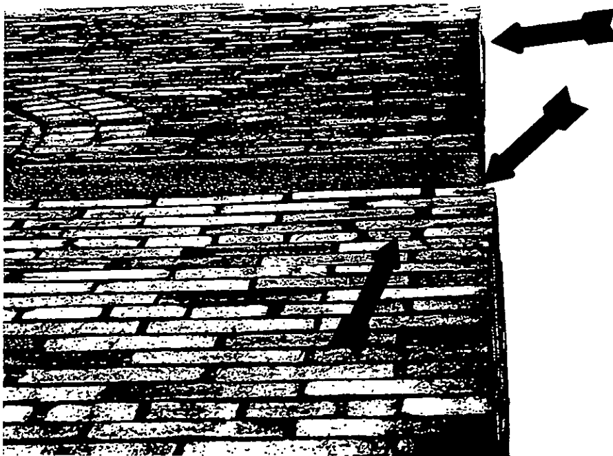
18. South Elevation At east corner bulkhead condition
