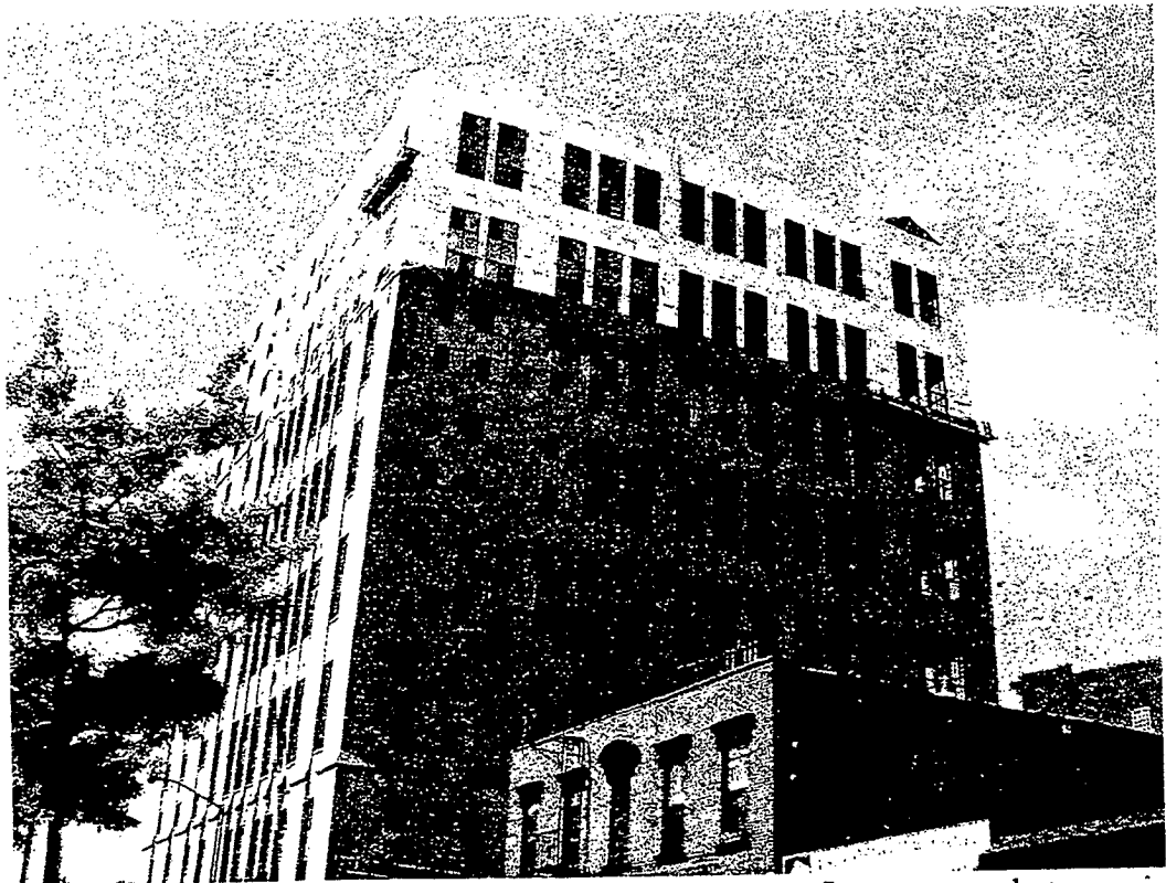
Picture #4 – North elevation on May 8, 2001, upper two floors are ready to receive GRFC cladding panels.
