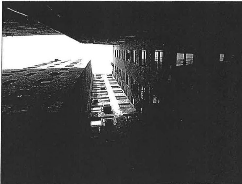
Photo 5 (taken 8/7/12) – Partial East Courtyard
