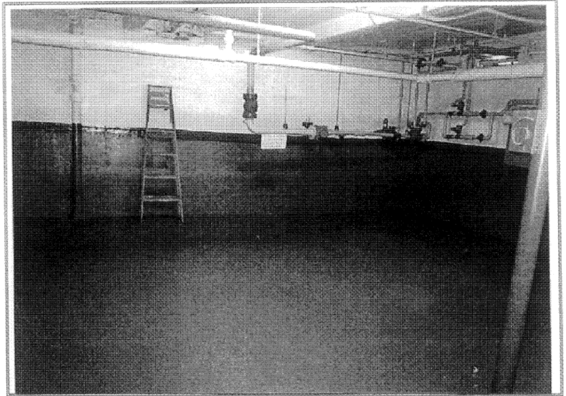
View of the main gas meter
