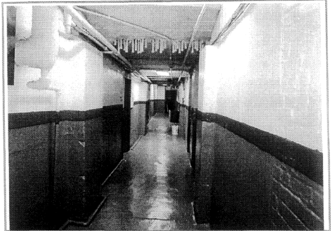
View of a typical hallway
