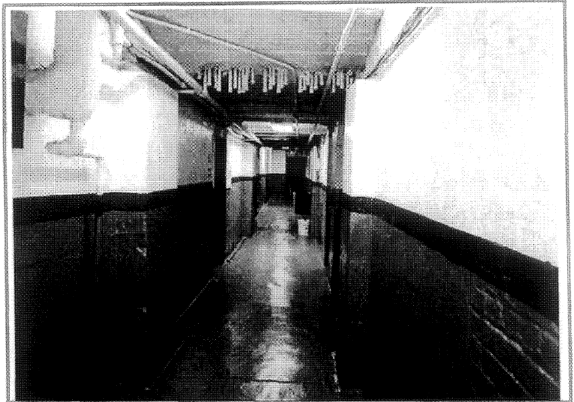
View of a typical hallway
