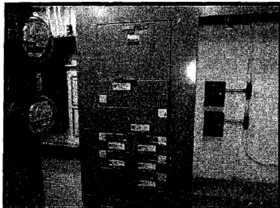
Figure 2.3.7 – Distribution Panels TYP.
