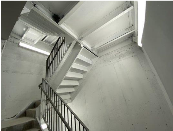
Over view of common stairwell; no susceptible materials and no damage observed on Floor 6 where minor gypsum board is found on the landing
