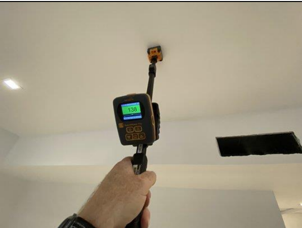
Typical MC in cellar ceilings; representative of 1 st floor unit; with no physical damages observed
