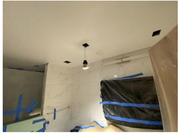
Overview of 1 st Floor Primary Bathroom; normal findings
