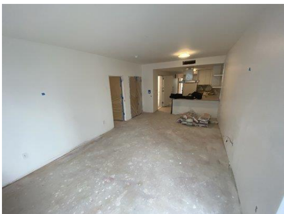
Overview of typical 5 th floor through 2 nd floor layout of the living room and kitchen
