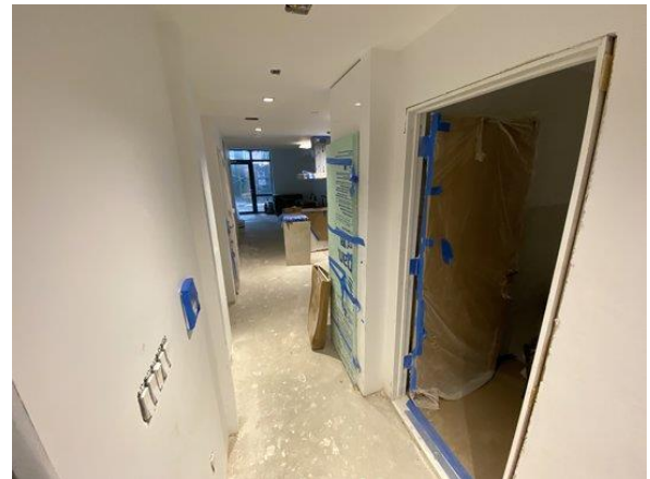
Overview of 1 st Floor unit from entry door
