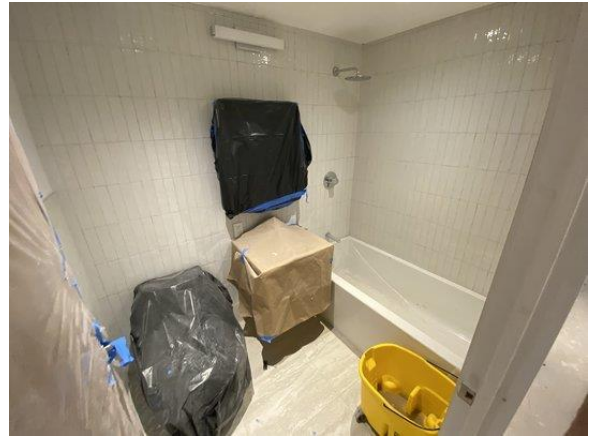
Typical Bathroom 2 layout from Floors 5 through 2; normal findings
