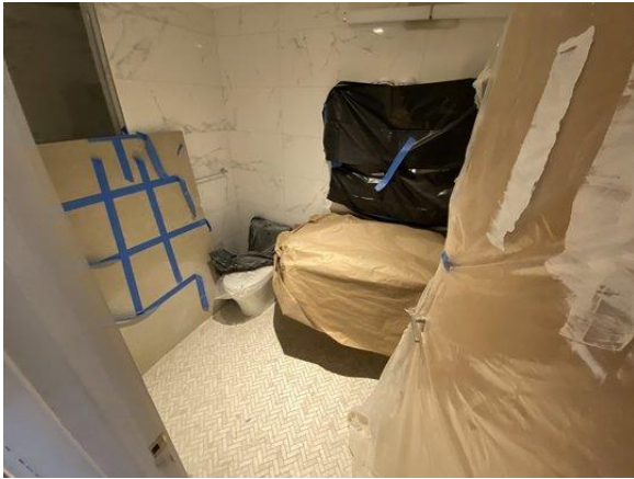
Typical Primary Bathroom layout from Floors 5 through 2; normal findings
