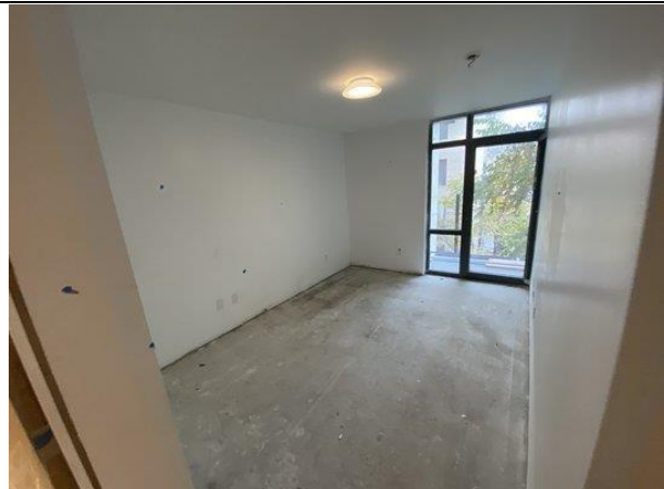
Typical Primary Bedroom layout at the NW corner from Floor 5 through 2; normal findings
