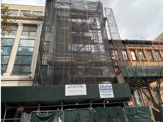
Overview of property from street
