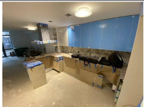
1 st Floor unit kitchen overview; normal findings; slight odor detected at left at top of cellar entry stairwell
