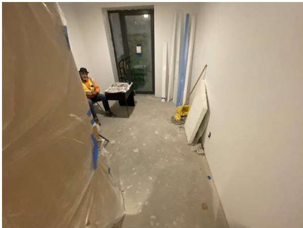
Front bedroom in 1 st Floor unit; normal findings
