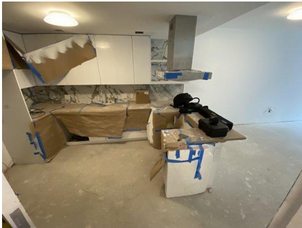
Typical kitchen layout and overview from Floor 5 through 2; normal findings
