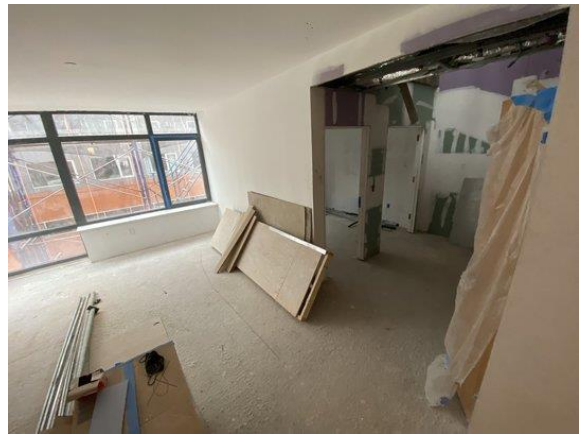
Overview of 6 th floor unit front living room and adjacent bedroom & bulkhead entry space
