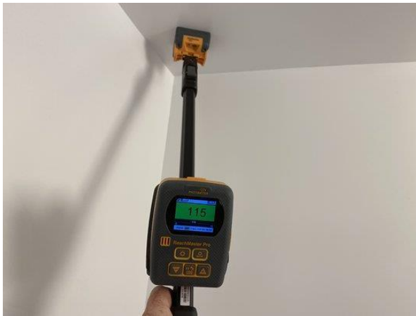
Verified to be dry; no damage related to water issues or microbial growth were observed
