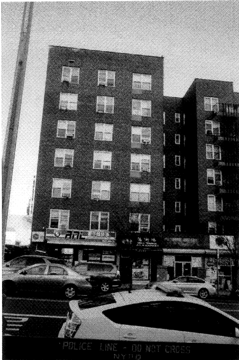
Figure 3: North End of West Elevation
