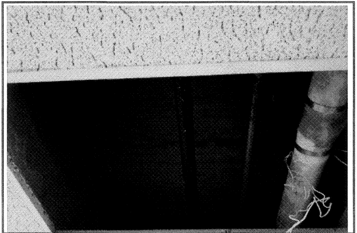
View above ceiling tiles
