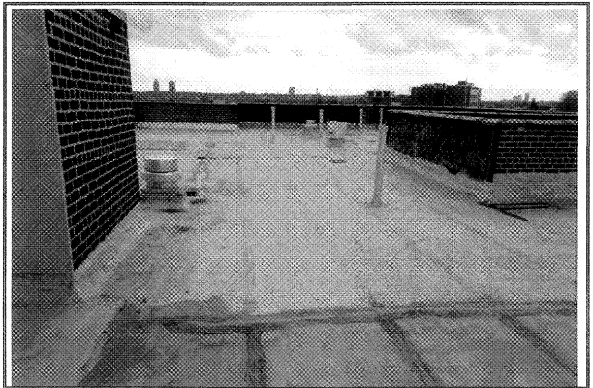
View of the roof
