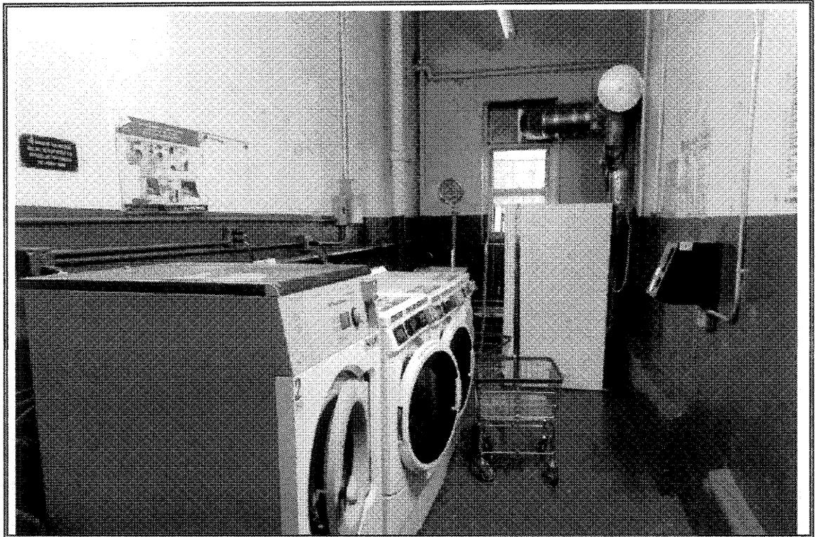
View of the laundry room
