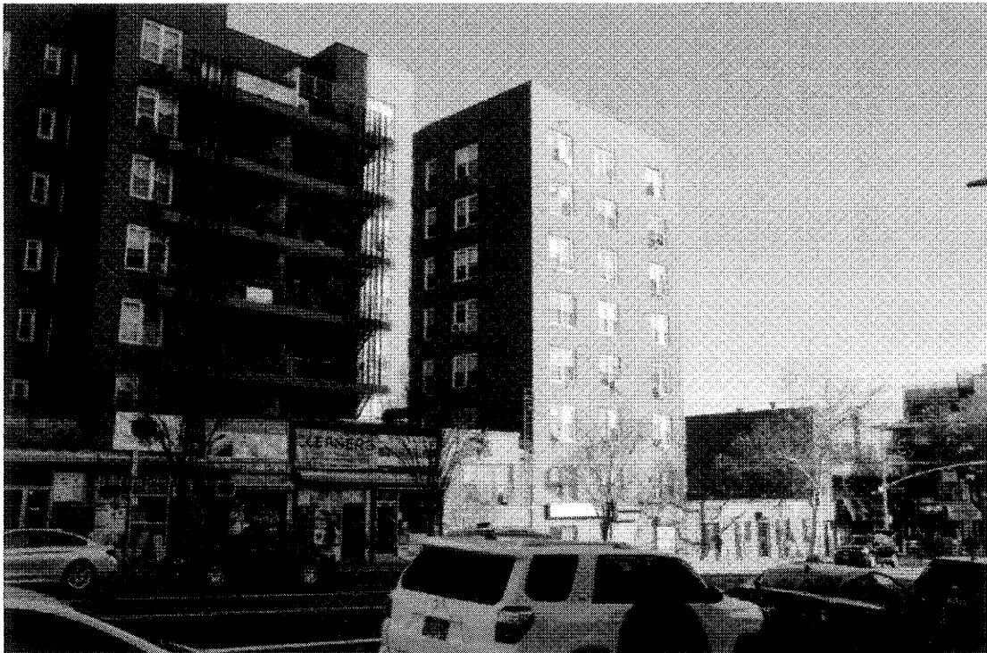
Figure 2: South End of West Elevation
