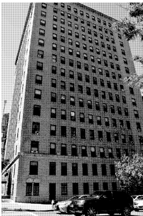
Photo #3: Exterior of building
