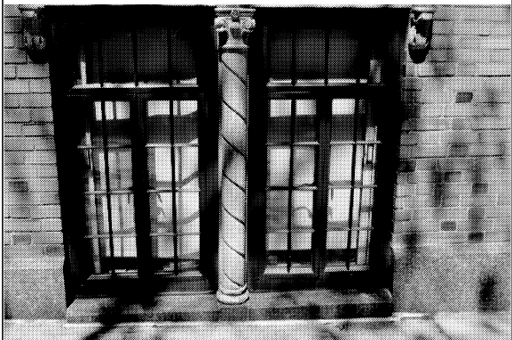
Photo #6: Typical windows
