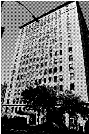
Photo #1: Exterior of building
