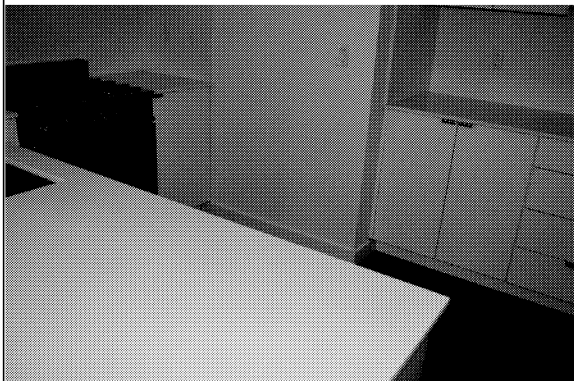
Photo #41: Typical renovated unit interior
