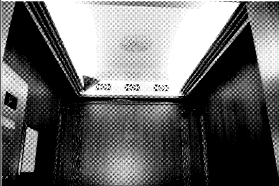
Photo #31: Elevator cab interior
