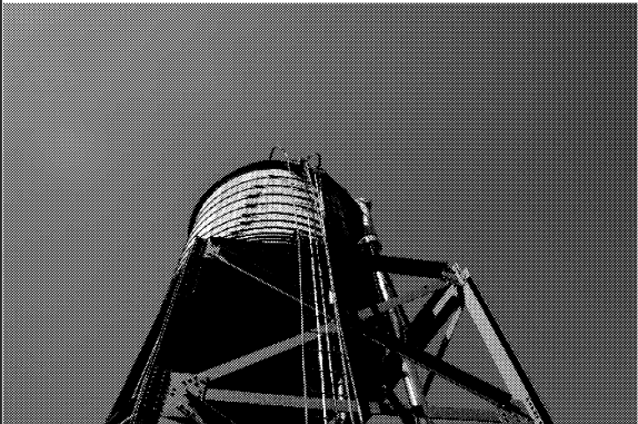
Photo #16: Domestic water storage tank
