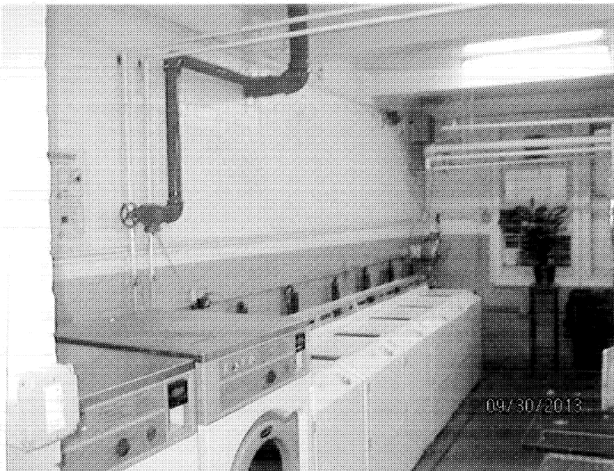
8. Basement laundry room looking north at bare, red sprinkler line..
