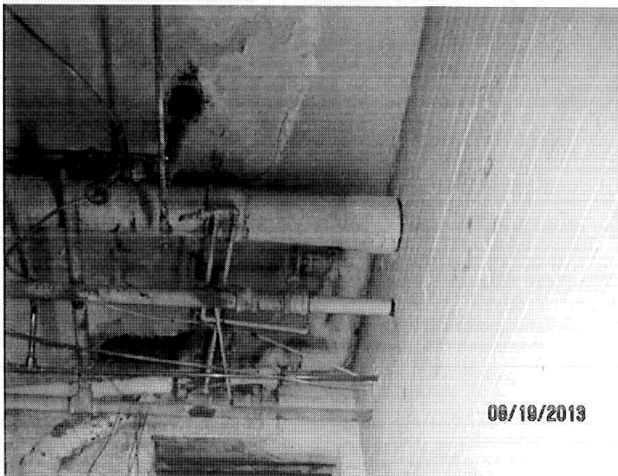
6. Basement boiler room ACM piping in the NE corner.
