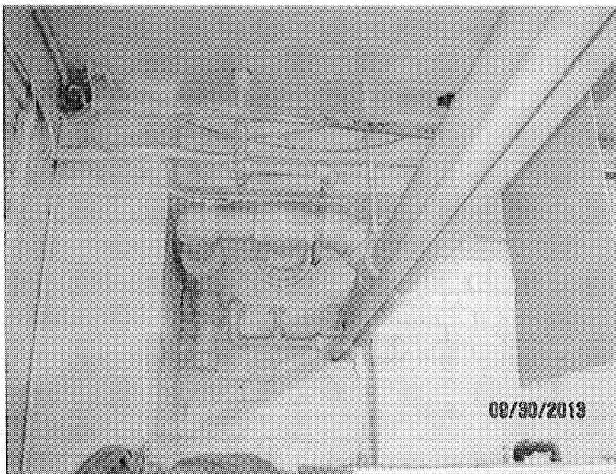
10. Looking east at bare heating pipes in the basement laundry room.
